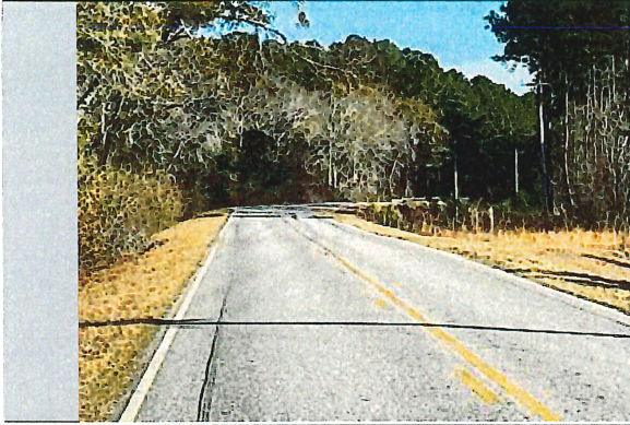
Photo 1. View of pavement at Bulloch County Line
