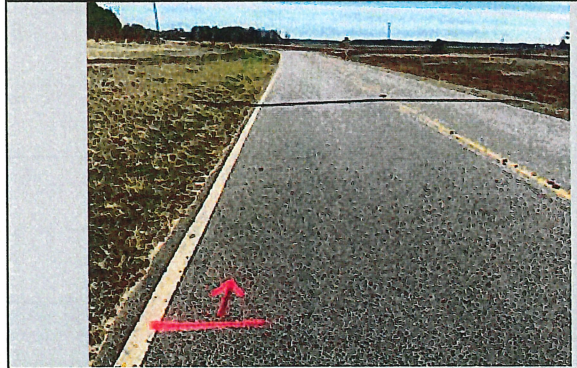
Photo 3. View of Evaluation Segment on East Side
