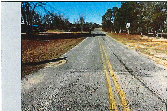
Photo 1. View of beginning of roadway segment @ SR 46.
