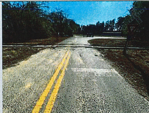
Photo 2. View of surface treatment near Railroad crossing.
