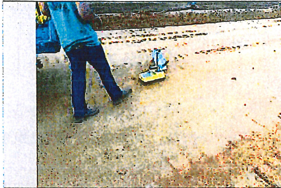
Photo 1. Density Test Was Performed on Subgrade - Pass
