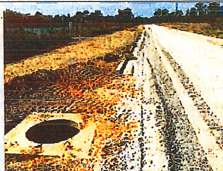
Photo 4. View of STMH awaiting proper protection to be installed.
