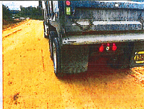
Photo 2. Proof Roll was Performed on Sub-grade
