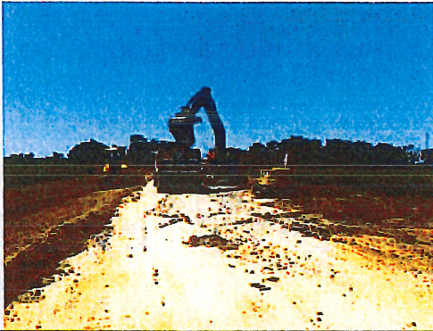
Photo 1. View of ongoing excavation operations.
