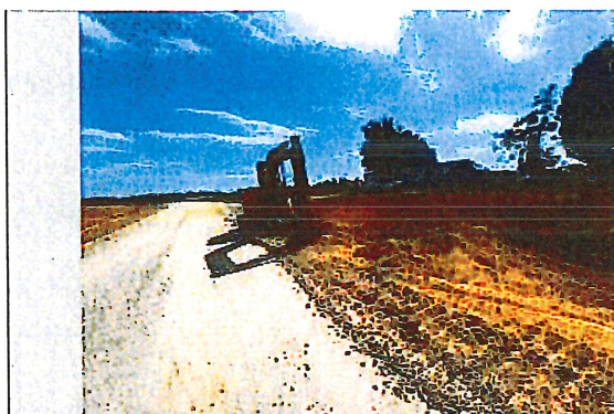
Photo 1. View of excavation operations on-going.
