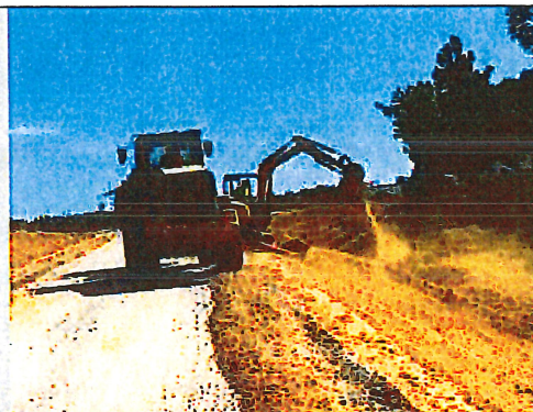
Photo 2. View of excavation operations on-going.
